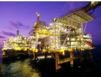
ConocoPhillips Bayu-Undan Operations & Maintenance Photograph courtesy of ConocoPhillips Australia Pty Ltd
