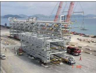
Assembly Yard Sattahip, Thailand
