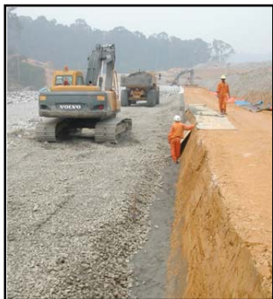
Namuk Tailings Dam, East Kalimantan
