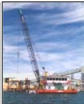
Bunbury Marine Piling, Western Australia
