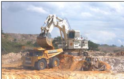
BBE Pit Coal Mining, Kalimantan
