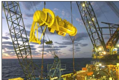
Java Constructor – Mid water arch installation
