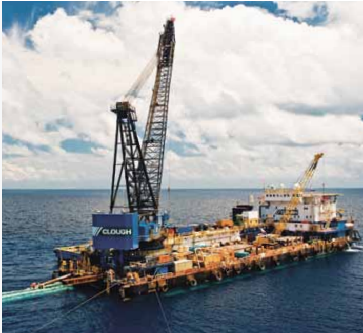
Java Constructor on ROIC Pipeline Installation Project
