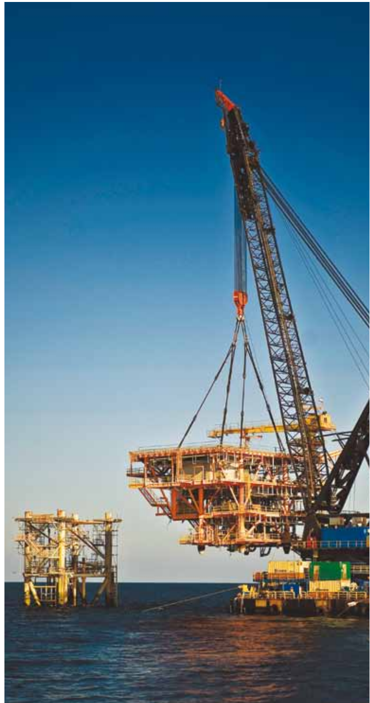
Clough's Java Constructor Derrick Pipelay Vessel installing the Montara topsides
