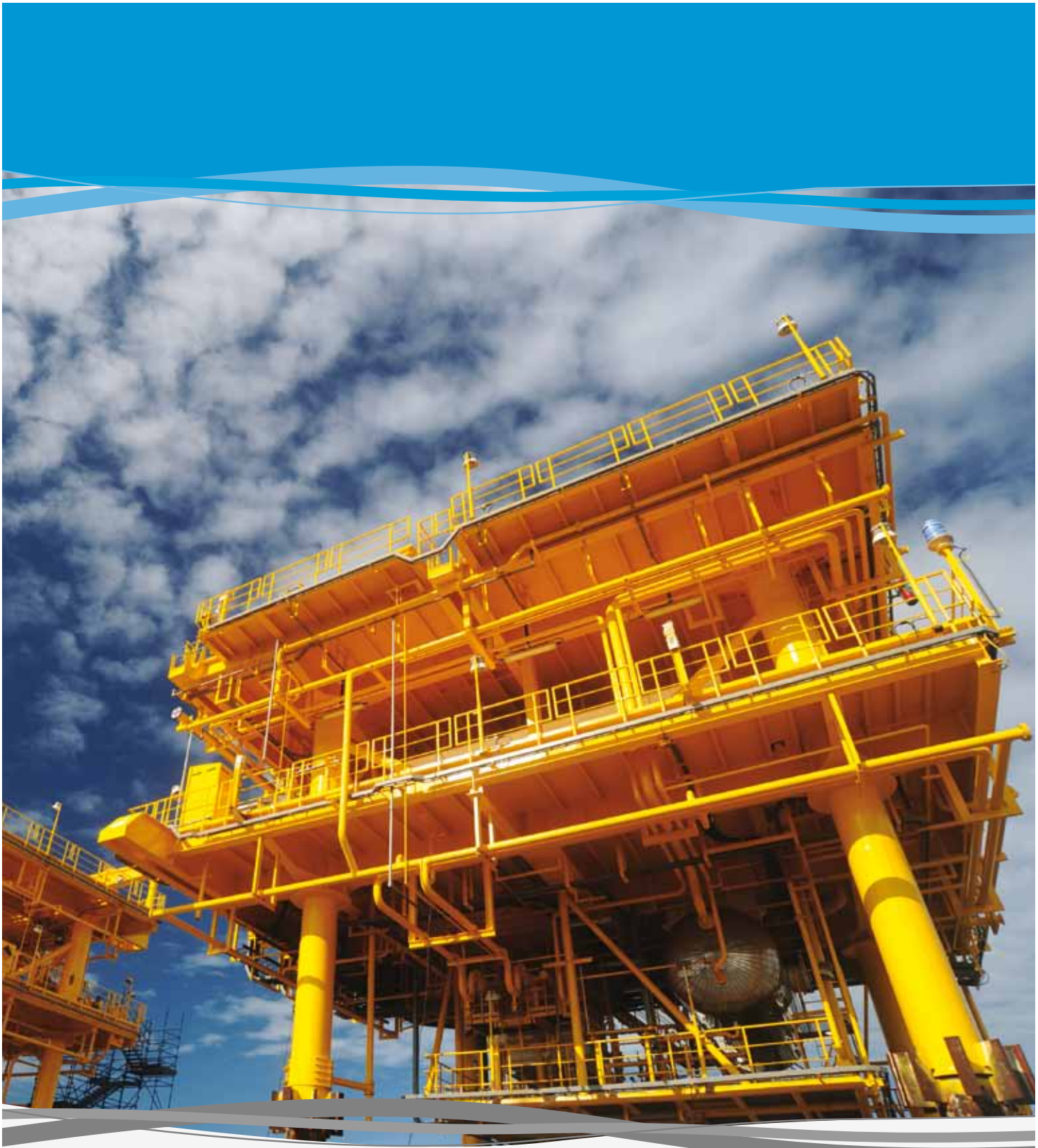
NuCoastal Bua Ban Field Development Topsides at Clough's Sattahip Fabrication Yard
